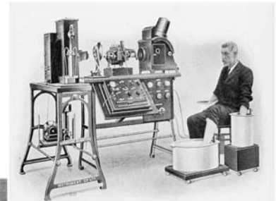
PHOTOGRAPH OF A COMPLETE ELECTROCARDIOGRAPH, SHOWING THE MANNER IN WHICH THE ELECTRODES ARE ATTACHED TO THE PATIENT. IN THIS CASE THE HANDS AND ONE FOOT BEING IMMERSED IN JARS OF SALT SOLUTION
